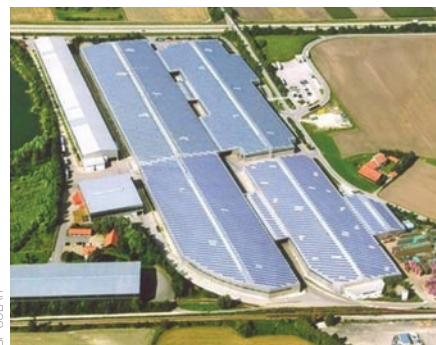
Germany has led the world in photovoltaic installations. Here a whole factory roof is covered with solar cells.
